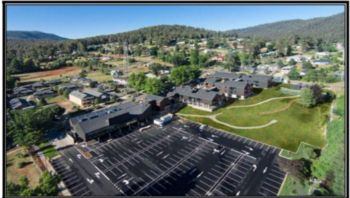
Figure 6.27: An aerial view of the rear of the Vibe Hotel, Marysville. 196
