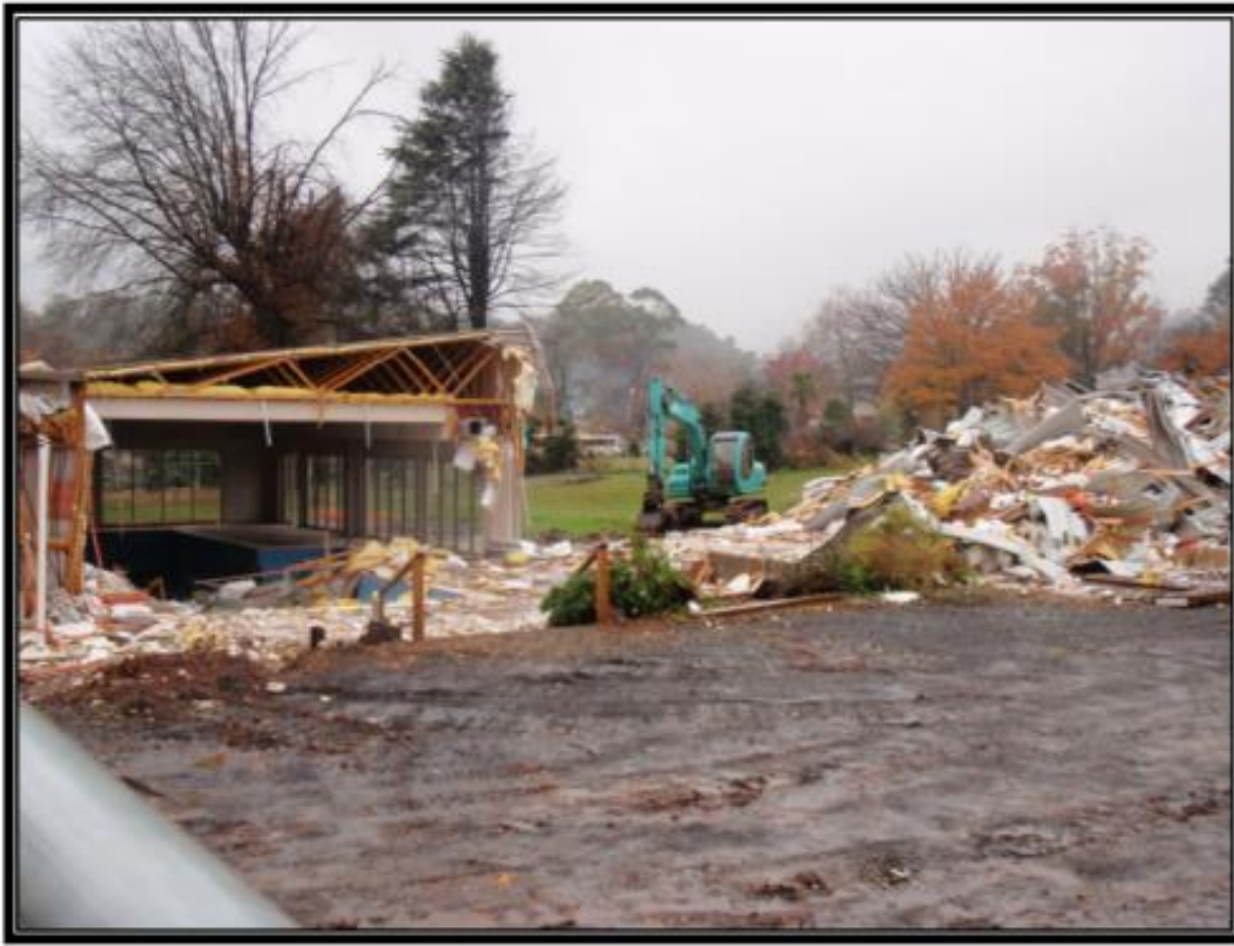
Figure 6.23: The rapid demolition of the Marysville indoor pool – 1/6/2013. 189
